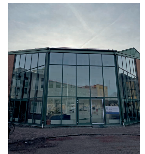
J. Detail of glass entrance and waiting room
