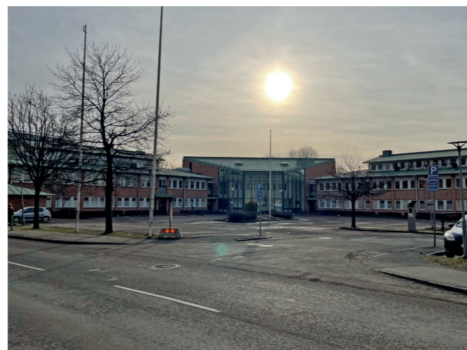
D. View towards property from the road
