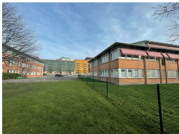
C. View towards property and grey parking lot
