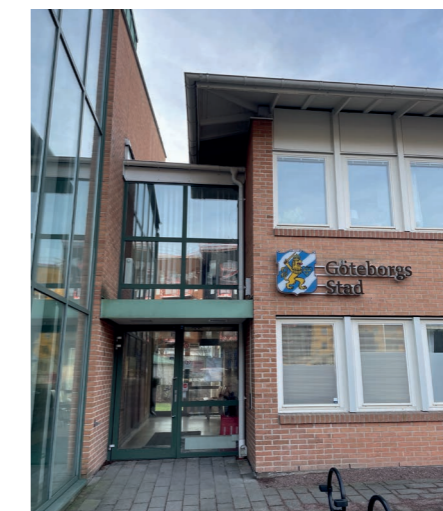
I. Detail of glass corridors connecting the three parts of the building
