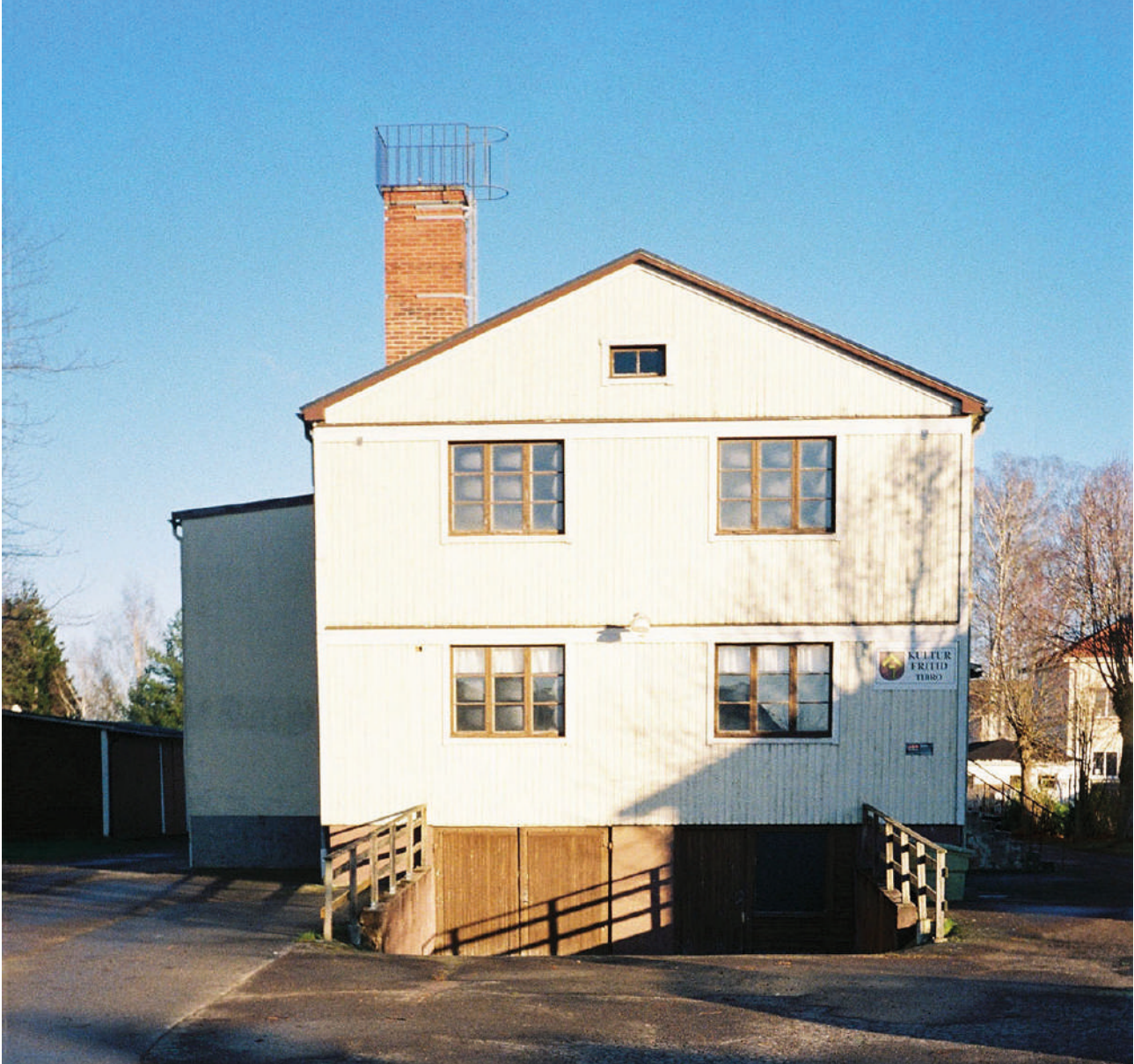
Former association building, Humlan
