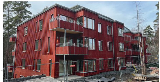
Low window sill height
