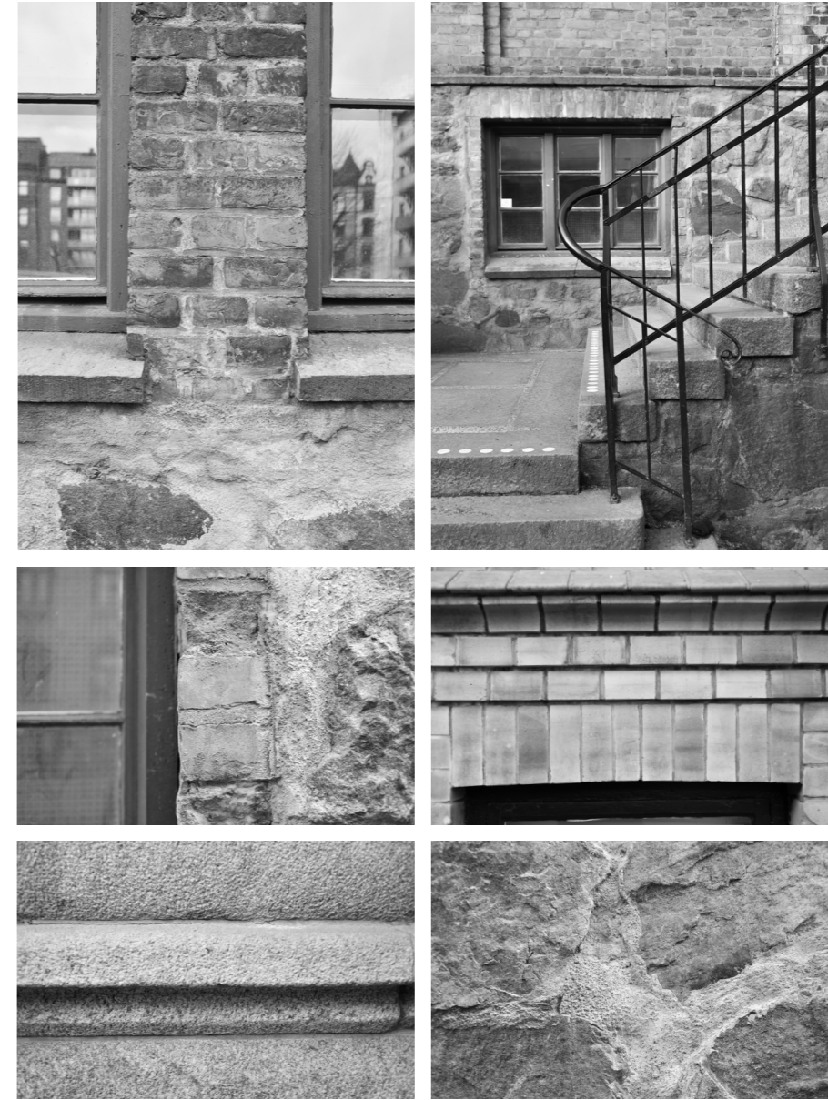
Photos of facade details of Viktoriahuset, built in stone, brick, and ironwork.
