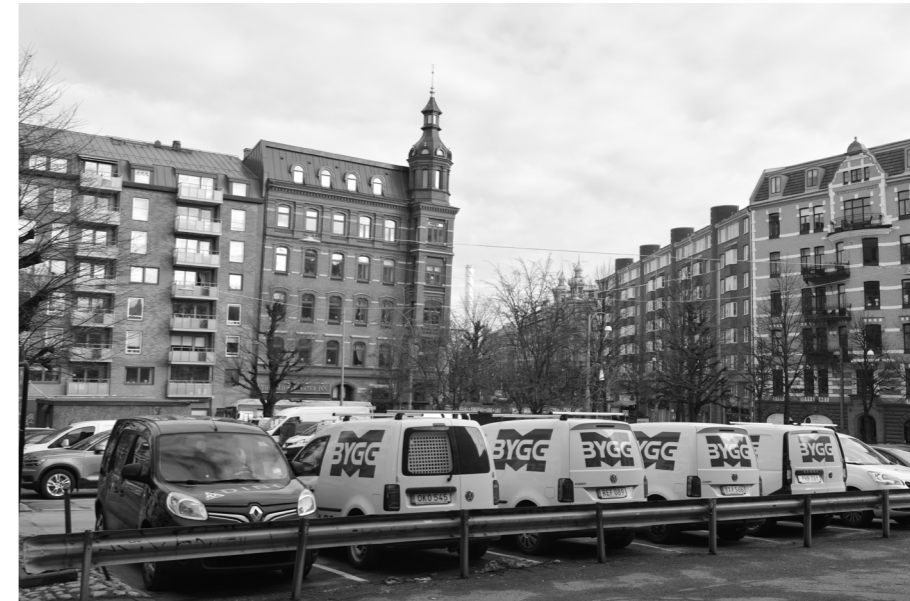
Upper photo: Nordhemsgatan and the different height of the buildings.
