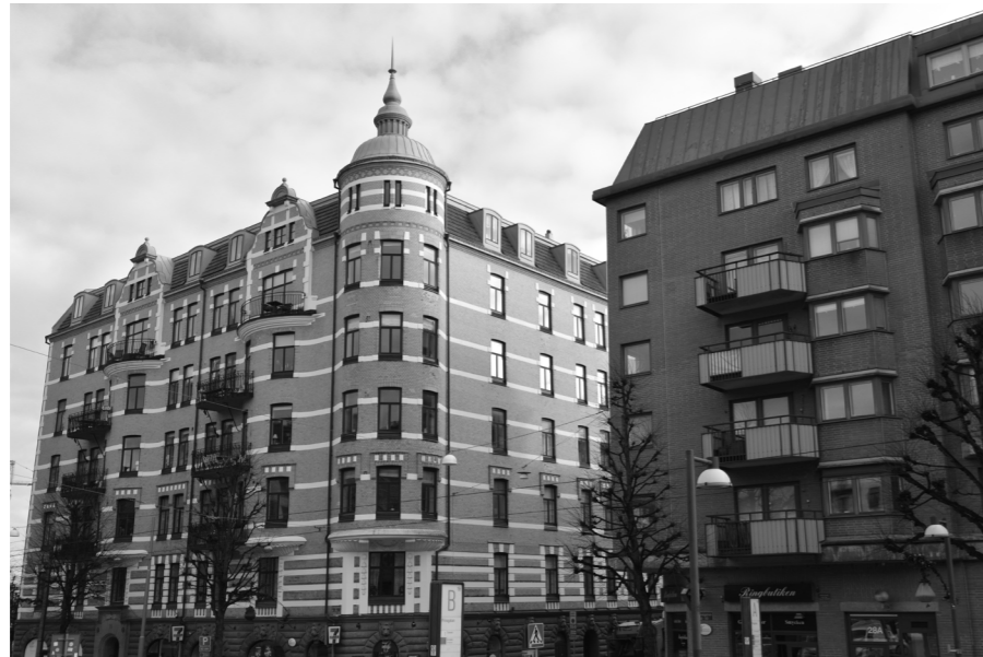
Upper photo: The north facade of Viktoriahuset, displaying strict organisation of windows and facade elements.
