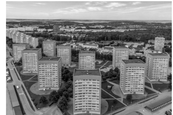
Figure 4.5: High rises, Västra Frölunda
