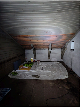
Figure 39. 16. Room without tie rods with wooden roof
