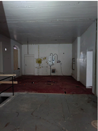
Figure 48. 24. Floor made of concrete, tiles, and metal hatches. Placement of power supply
