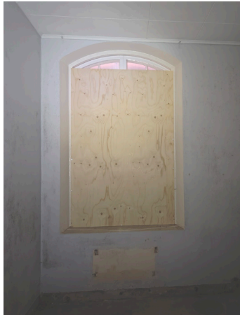
Figure 45. 21. Window and traces after radiator
