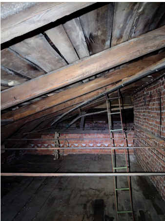
Figure 40. 17. Roof structure and visible bricks
