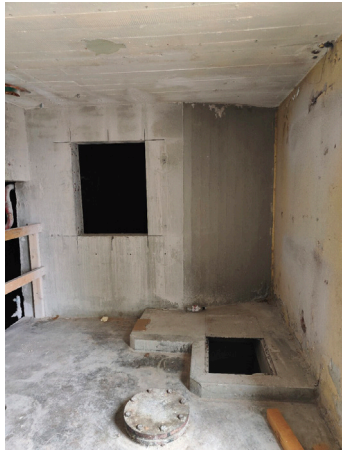
Figure 43. 19. Cisterns and an opening in the floor, surface layers in poor conditions
