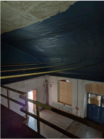
Figure 38. 15. View of entrance floor
