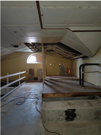
Figure 36. 13. Inner ceiling and upper part of cisterns
