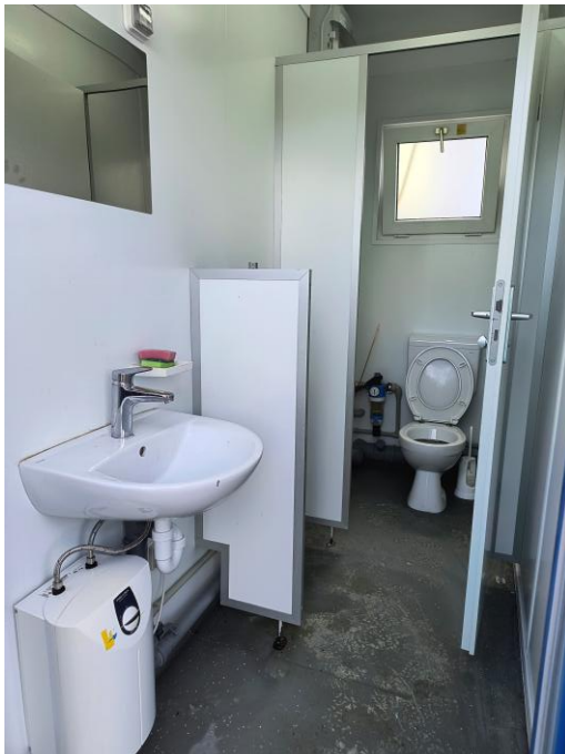
Figure 11: Men's toilet in sanitary container on site 2. (Picture taken by the author)
