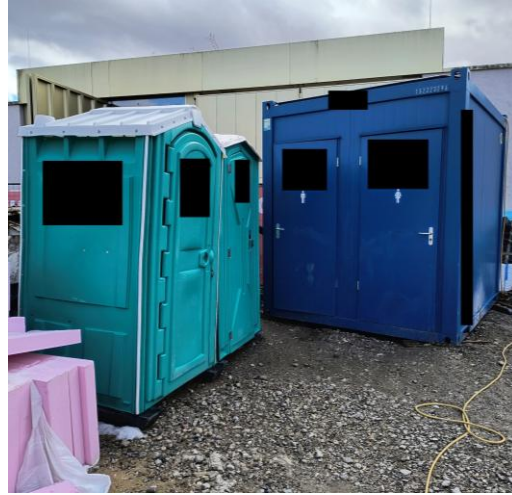
Figure 10: Sanitary facilities on site 2. (Picture taken by the author)
