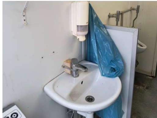
Figure 6: Sink in the sanitary container on site 1. (Picture taken by the author)
