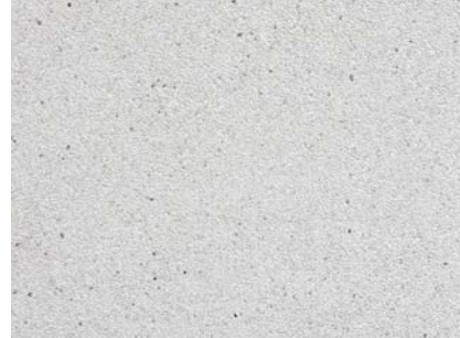
Figure 42. Concrete with exposed aggregate. (Finja)
