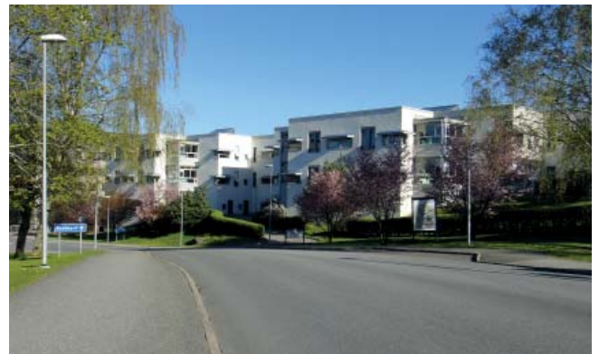
Figure 30. The psychiatric clinic at Östra Sjukhuset Photo taken by the author
