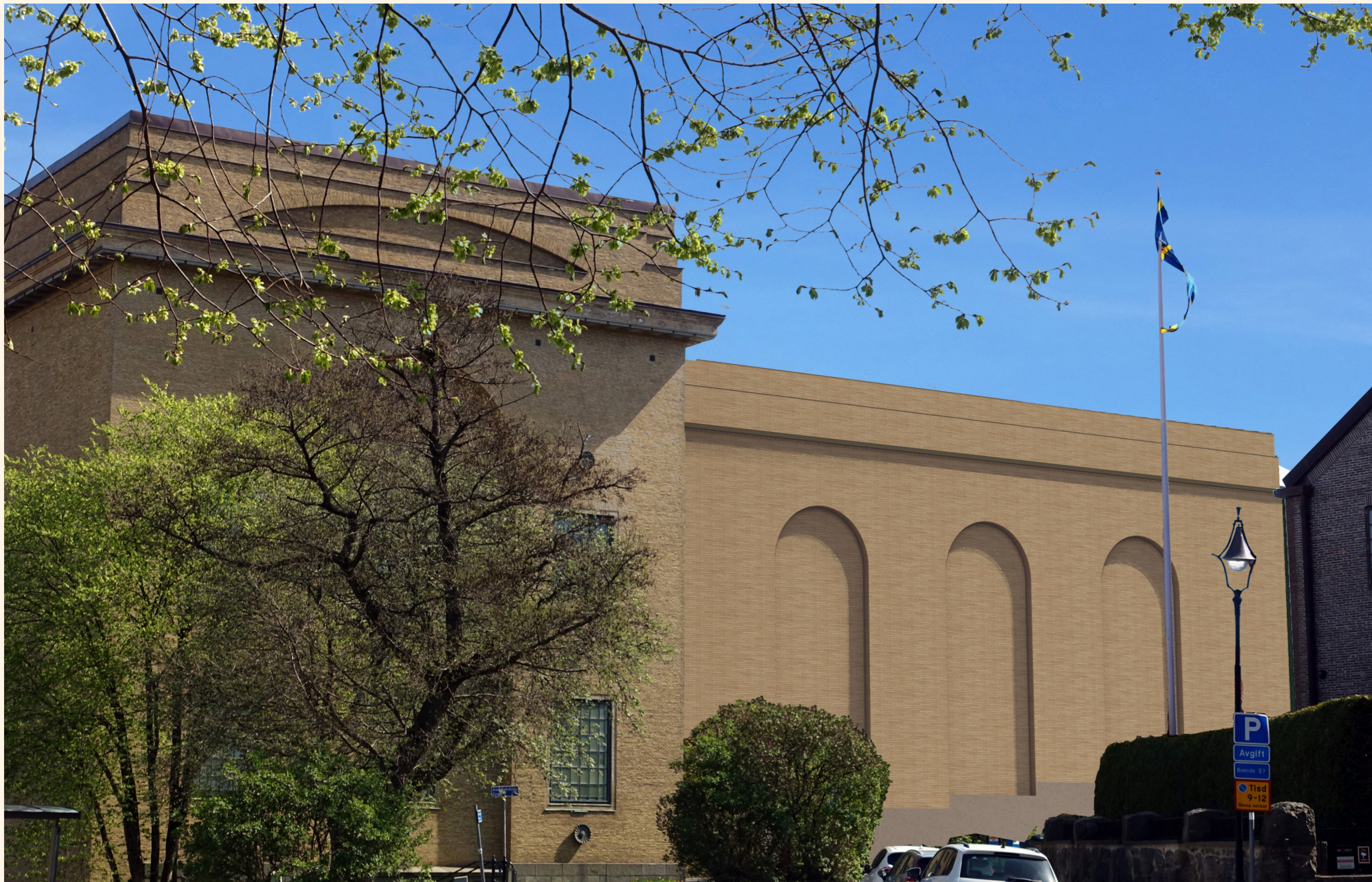
View of the extension from Ekmansgatan
