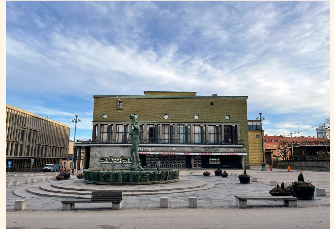
Figure 38: The City Theatre by Carl Bergsten, completed in 1934
