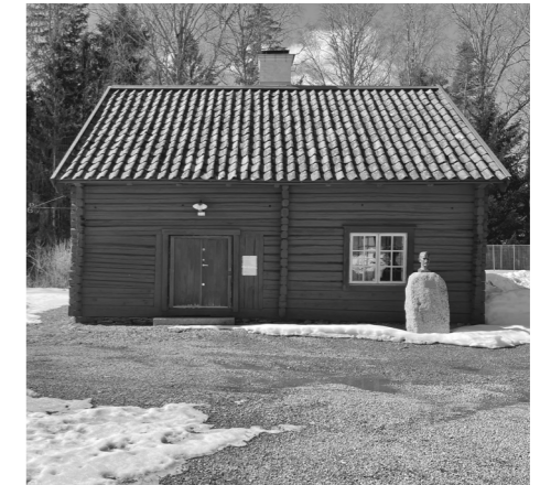
Log timber shed.
