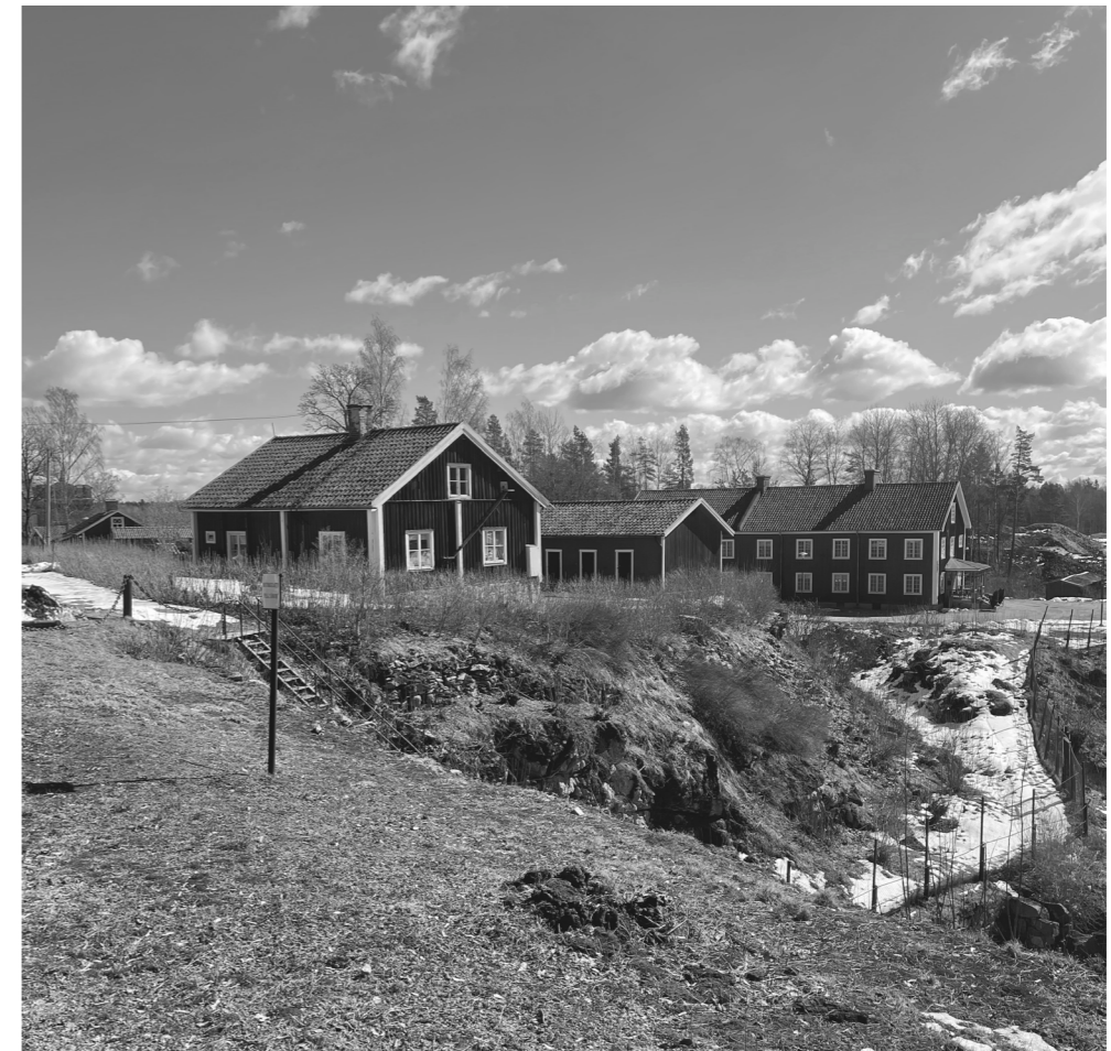
Scattered buildings at Sala Silvermine.
