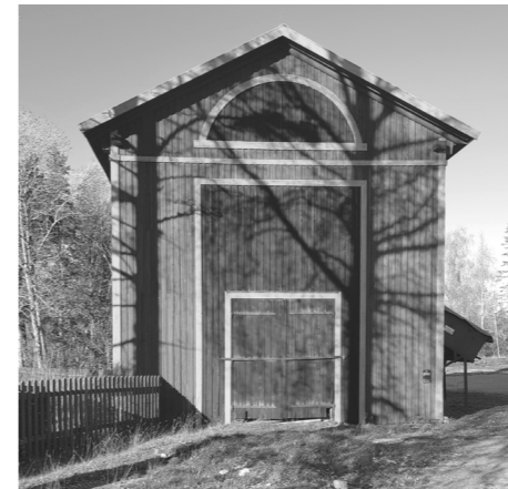
Headframe building, Wilhelm's mine.
