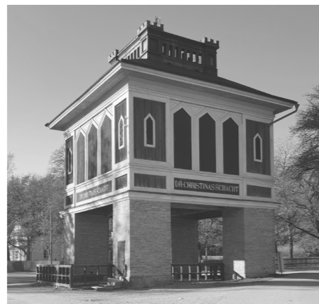
Headframe building, Queen Christina's shaft.
