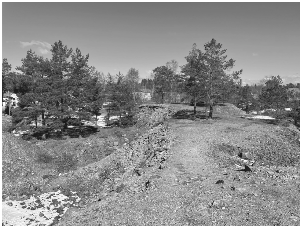
From above the piles of warp stone.
