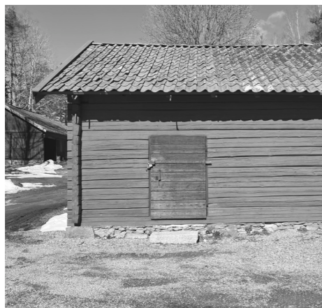
Log timber shed.
