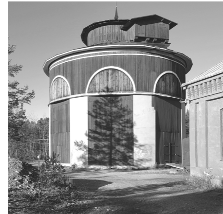
Headframe building, Karl XI's shaft.
