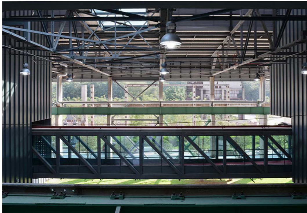
Figure 20: The linked bridges between the new added volumes.
