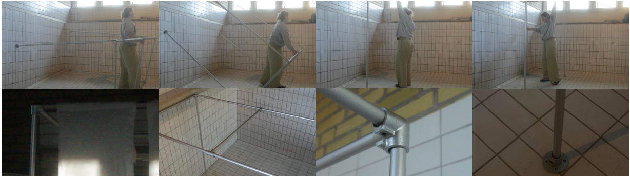
Installation of the construction.
