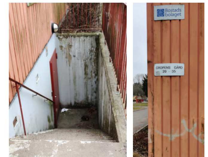
Figure (48) Basement where current laundry rooms is located
