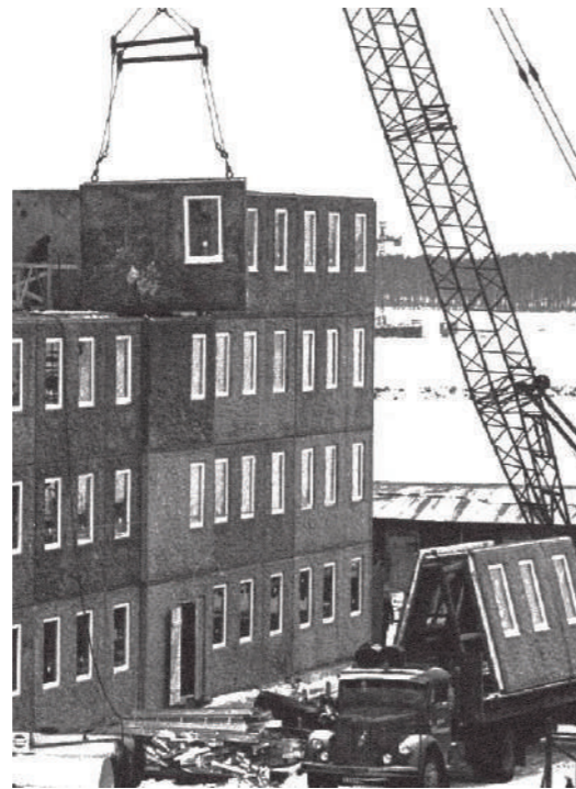
Figure (2) Stenberg Ohlson and Skarnes Skarne 66 during construction
