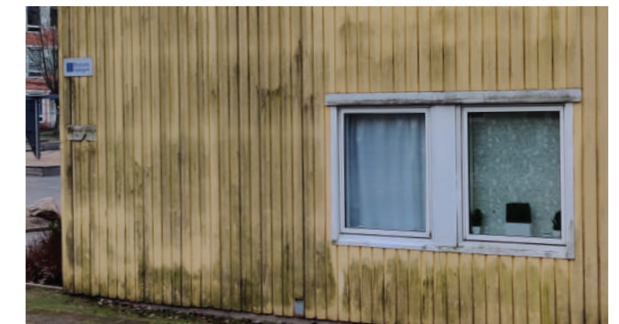
Figure (47) Facade condition
