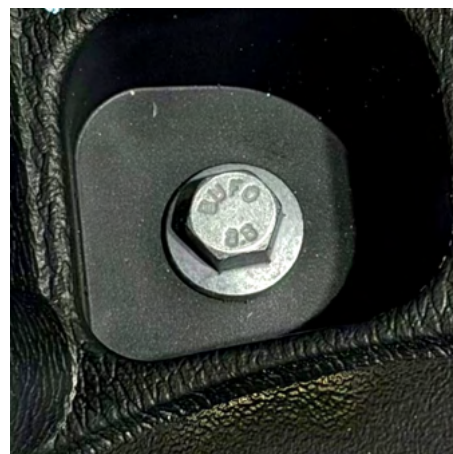
(b) Close-up of physical joint.
