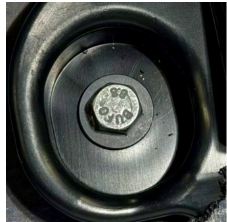
(b) Close-up of physical joint.
