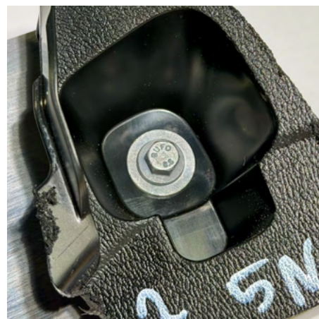
(b) Close-up of physical joint.
