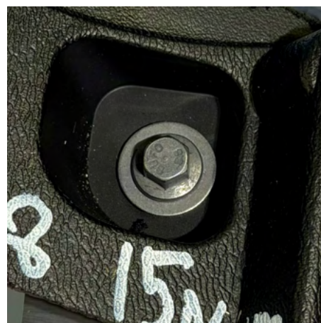
(b) Close-up of physical joint.
