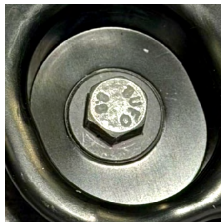
(b) Close-up of physical joint.
