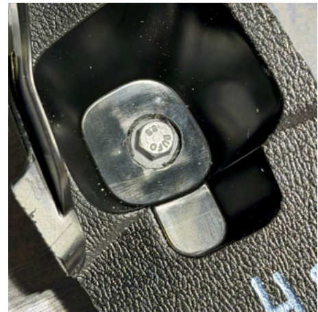
(b) Close-up of physical joint.
