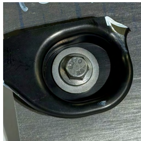
(b) Close-up of physical joint.
