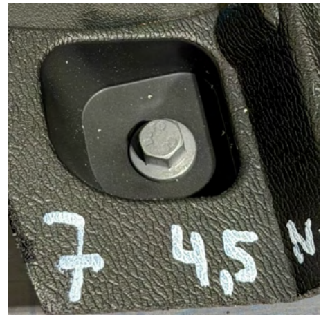
(b) Close-up of physical joint.
