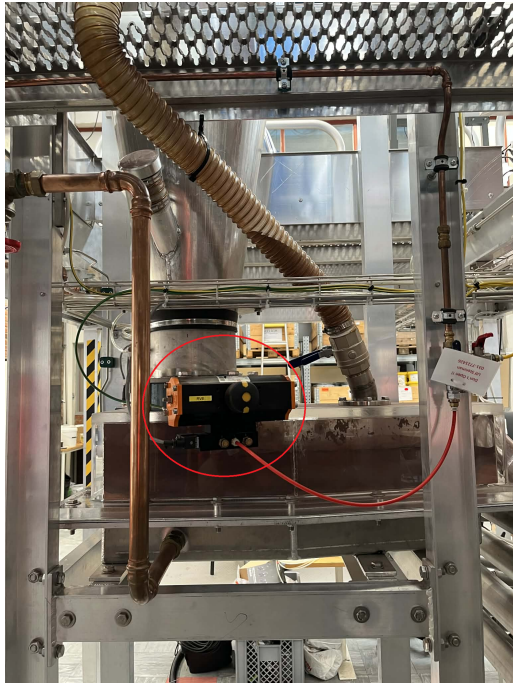
(a) Circulation valve at the loop seal.
