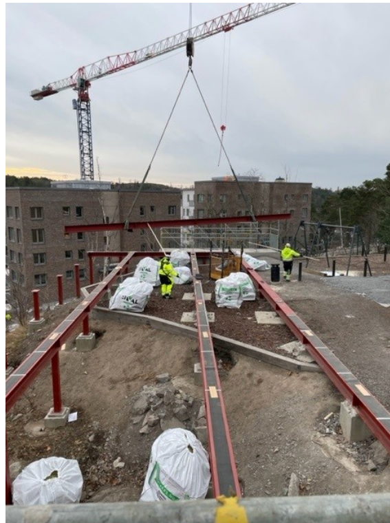
Figure 4.2: Picture from the dismantlement of the preschool. Source: Rival.
