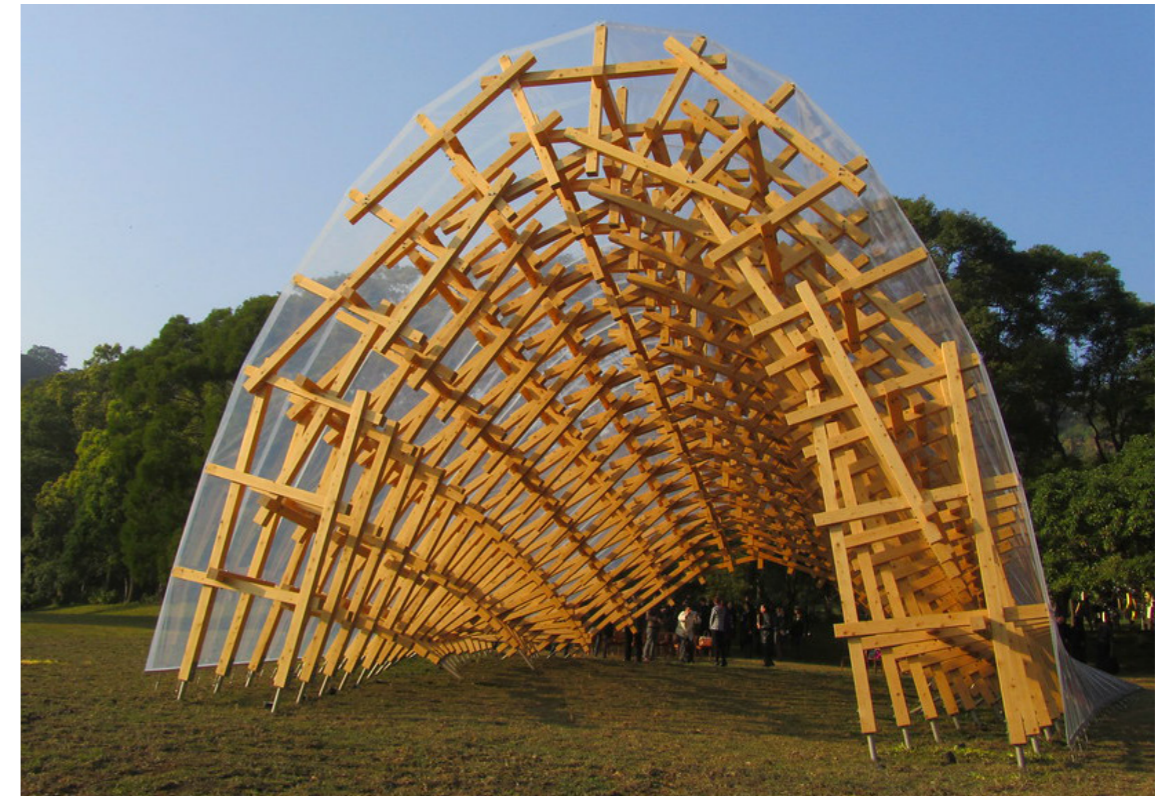
Image 2: Pavillion by Kengo Kuma using wood and flouropolymer membrane.(準建築人手札網站 Forgemind ArchiMedia, 2015)
