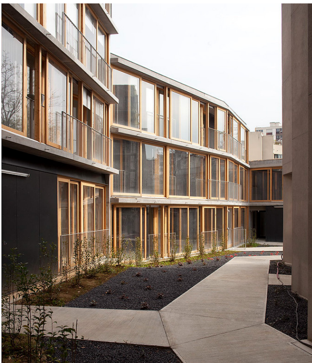
Pic.19: View of the apartments (Guillaume, 2013)
