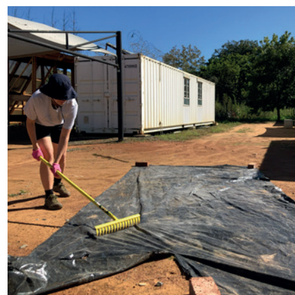
The process of perforation of reused plastic
