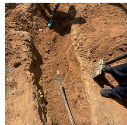
The digging of the ground around the pipe
