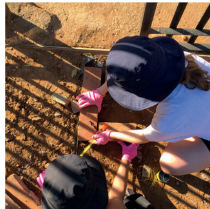
The placement of the first bricks
