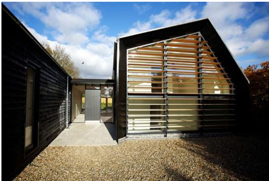
Figur 2.2. Bilden visar horisontella lameller. Copyright of Nationwide Louvre Company. (Nationwide Louvre Company, 2019)
