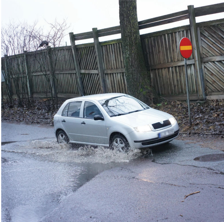
Fig. 27+28: Photos of Neptungatan after heavier rain, February 2025
