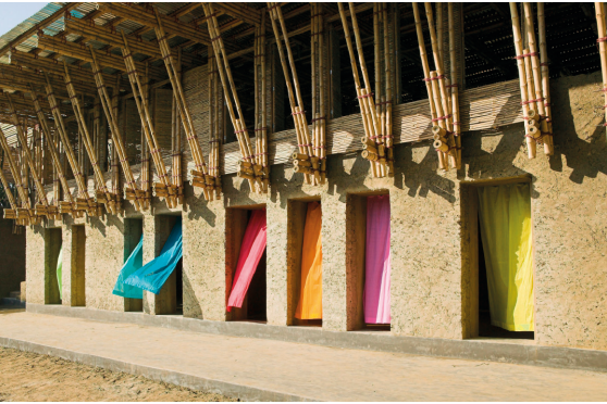
Figure 11. Cob wall under construction at METI School in Bangladesh (top) and finished cob wall at METI School (bottom). Photos ©Kurt Hoerbst
