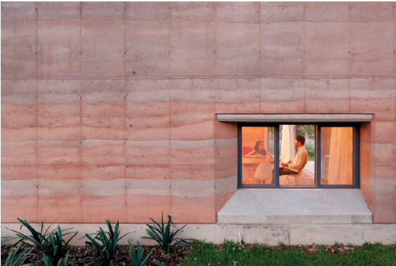
Figure 9. Rammed earth wall at Ajijic House. Photo © Iwan Baan
