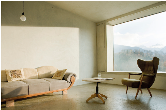
Figure 25. Interior featuring clay plastered walls and rammed earth flooring. Photo © Beat Bühler
