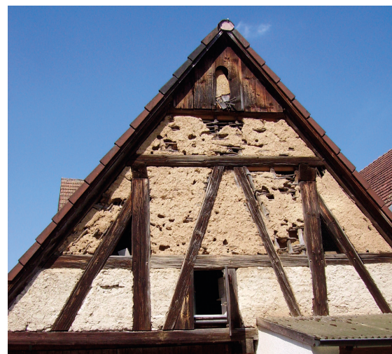
Figure 13. Traditional wattle and daub infill in timber framing in Heiligenstadt, Germany. Photo by Immanuel Giel.
