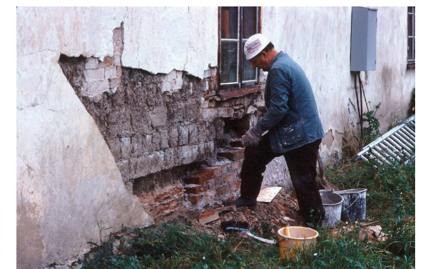
Figure 7. Exposed mudbricks during Svalbo's renovation. Image retrieved from Svalbo (n.d.).
