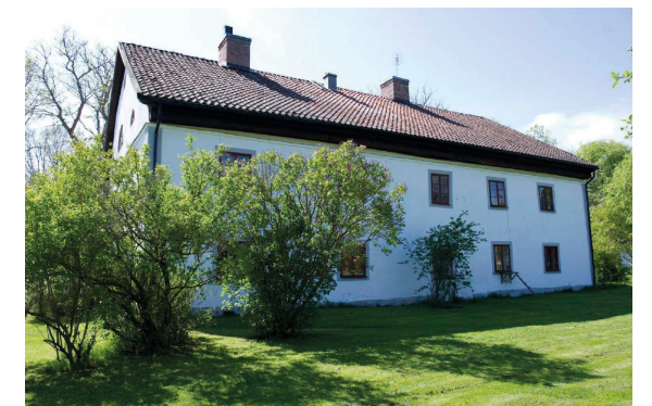
Figure 6. Svalbo is a building constructed with sun-dried clay bricks in the second half of the 18th century in Järle, 30 km north of Örebro. Image retrieved from Svalbo (n.d.).
