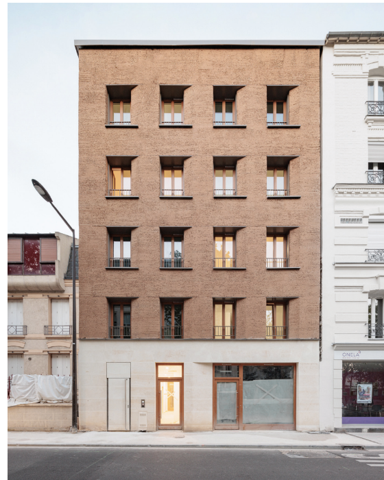
Figure 30. Photo of the facade towards the street. Photo © Salem Mostefaoui
