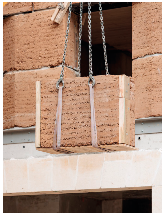
Figure 31. Prefabricated rammed earth elements during construction. Photo © François Baudry
