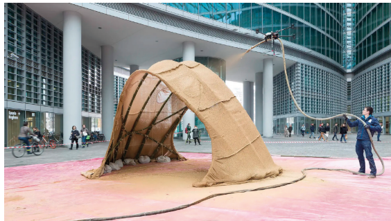
Figure 17. Drone spraying earth material on a textile formwork by MuDD architects. Photo © NAARO
