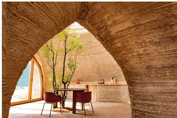
Figure 19. 3D printed earth house prototype - TECLA project. Photo © Iago Corazza
