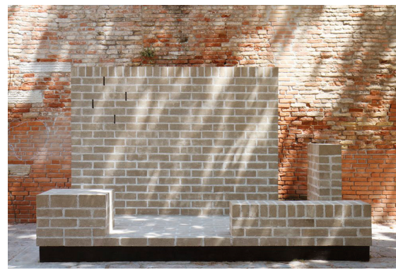
Figure 12. Adobe production in Madagascar. Photo © Pierre-Yves Babelon (top) and Compressed Earth Blocks installation at Venice Architecture Biennale 2016. Photo © Samuel Dématraz (bottom)
