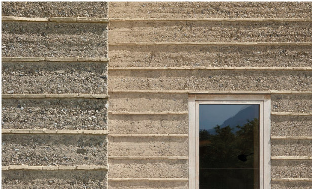
Figure 23. Detail image of the facade with protruding tiles as erosion checks. Photo © Beat Bühler
