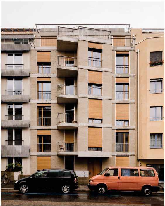
Figure 28. Exterior view from the street. Photo © Daisuke Hirabayashi
