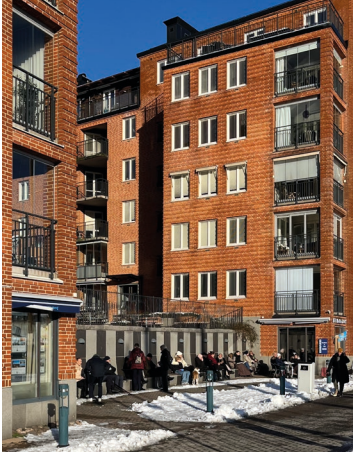
Fig. 3 The interior program is parking and there is no transparency or permeability. But the frontage afford interactivity either way because of the frontage design with a setback allowing for seating and enjoying.
