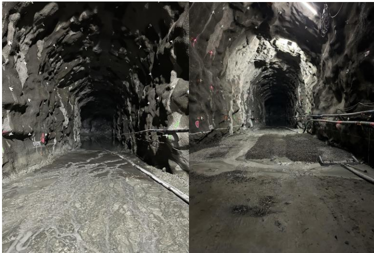
Figures 13 and 14. Sedimentation pond in tunnel ST-205.
