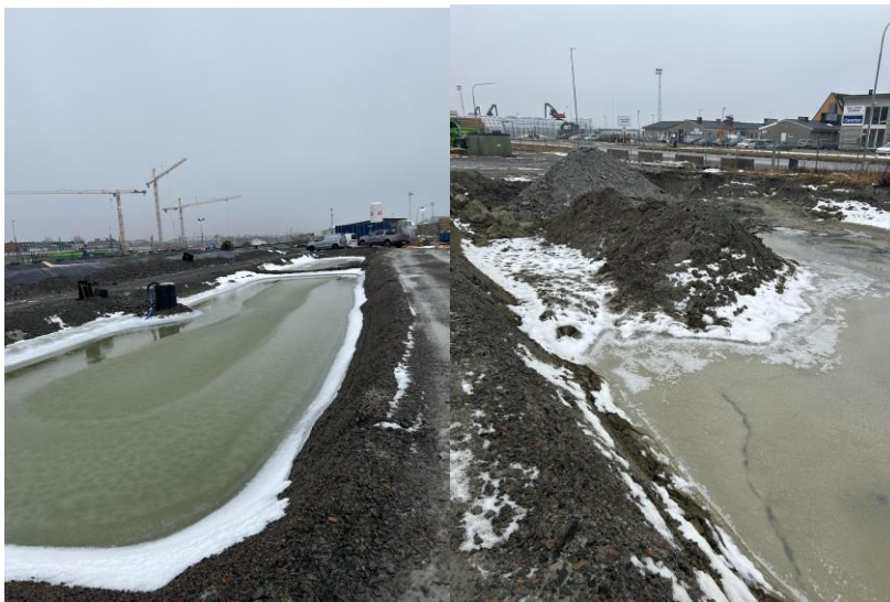
Figure 40 and 41. Sediment basins and sediment piles
