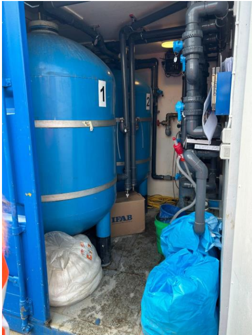
Figure 46. Active carbon filter and ion exchange filter
