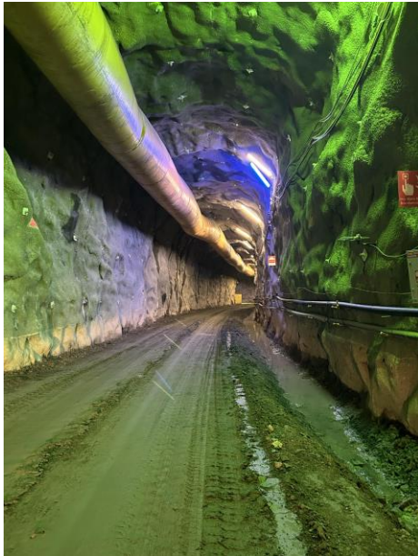
Figure 12. Ditches in the service tunnel (ST-101) for removal of particles through sedimentation.
