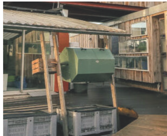
Fig.4.8. Compost Toilets (De Ceuvel, n.d.)
