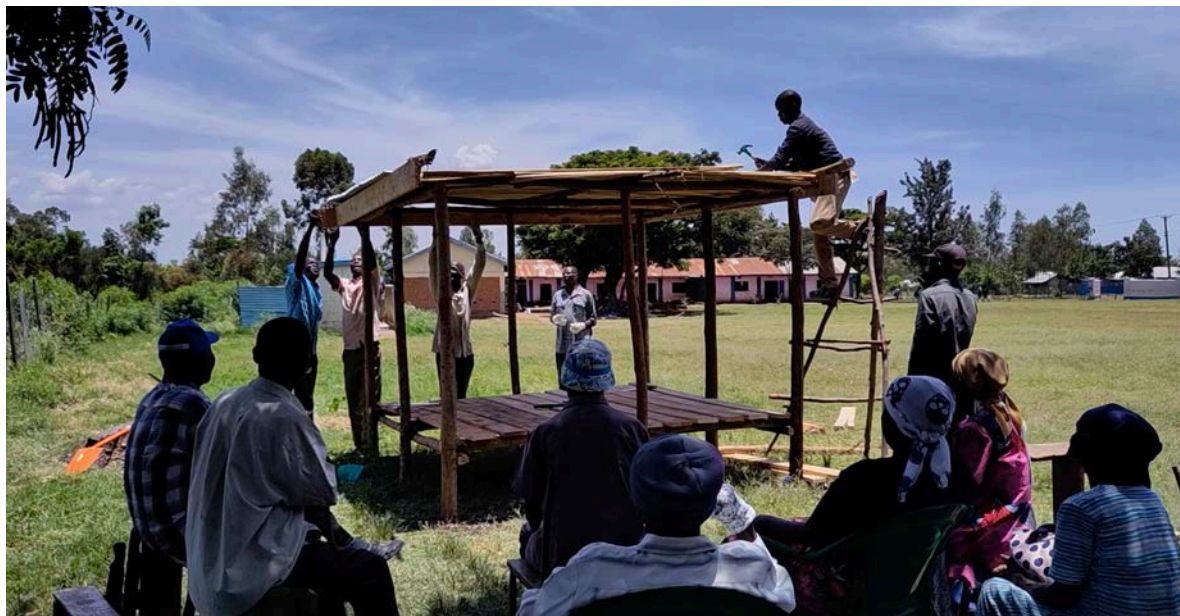
Figure 32: Members of the community watching their fellows build the prototype
