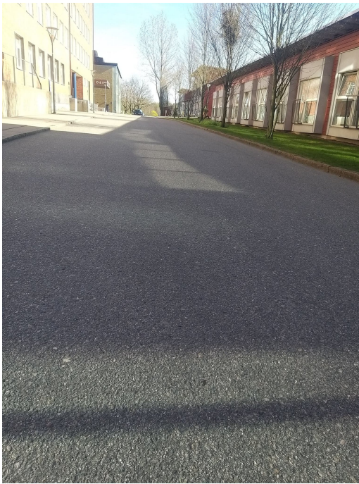
Figure B.5: Site 5 Pedestrian road 57.687979 N, 11.977886 E
