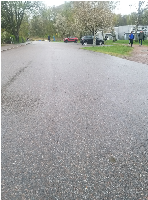
Figure B.6: Site 6 Pedestrian road 57.685060 N, 11.980295 E
