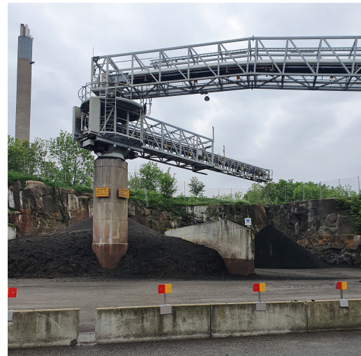
(b) Dewatered sludge storage
