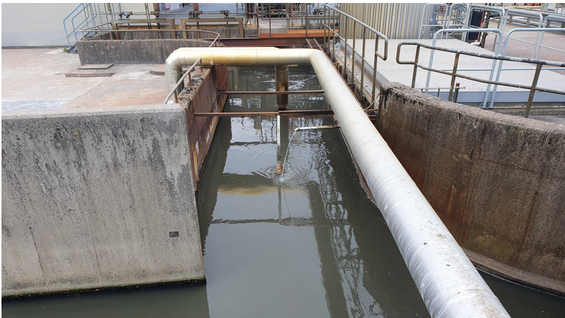
(b) Addition of \text{FeSO}_4 at Rya WWTP before the AS basins.
