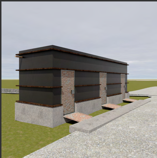
Fig. 102 Service node first stage of decay.
