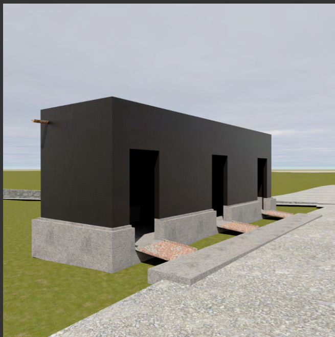
Fig. 103 Service node second stage of decay.
