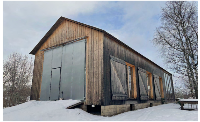
Fig. 24 Exterior of Atelje Södersvik. Untreated panel giving short term decay.
