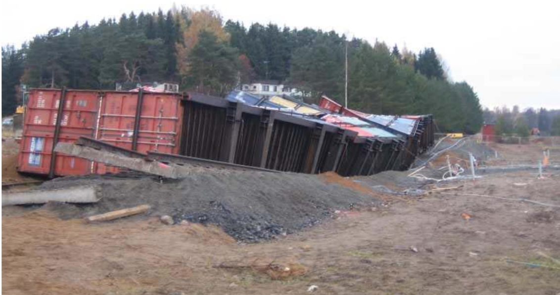
Figure 3.6: Photo taken at the site after failure of the embankment (Lehtonen, 2011).
