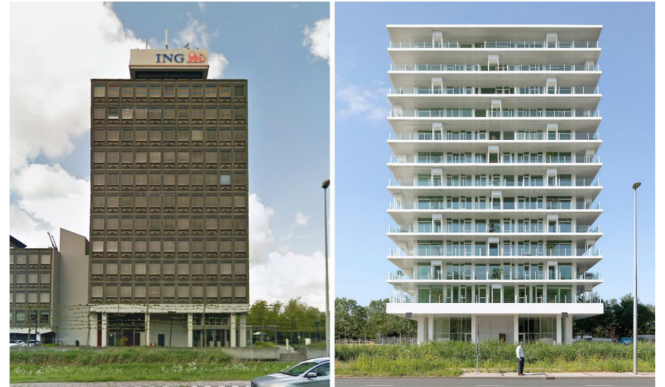
Figures 15a–b. Former ING bank remodelled into a residential building in Amsterdam by Elephant. Front gardens and elevators are incorporated into the façade.
