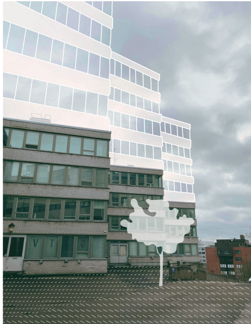
Figure 21. The guiding principle for building over has been to respect the integrity of the original structure. Here, an imagined addition to Hyvlerivägen 18 reflects the form and character of the existing volume.
