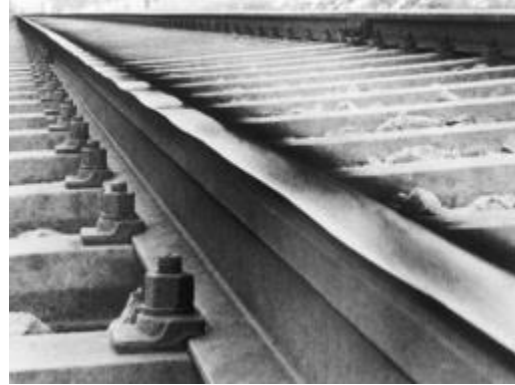
Figure 10: Long-pitch corrugation (from [29])
