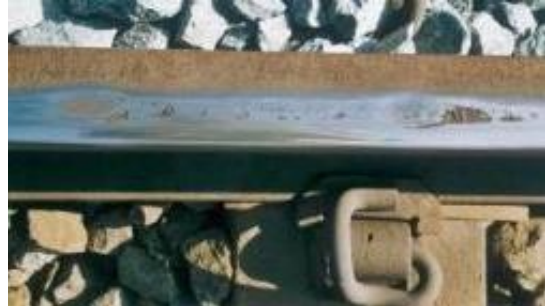
Figure 5: Wheel burns (code 2252) (from [29])
