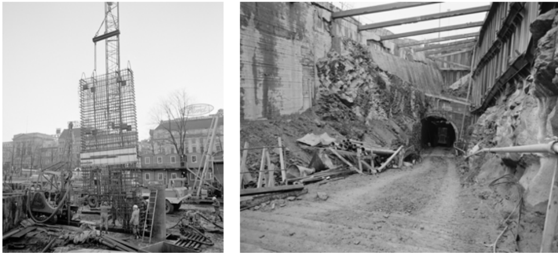
Figure 2.5: Construction of Studenterlunden in Oslo, Norway (Rude, 1972) (Rude, 1975).
