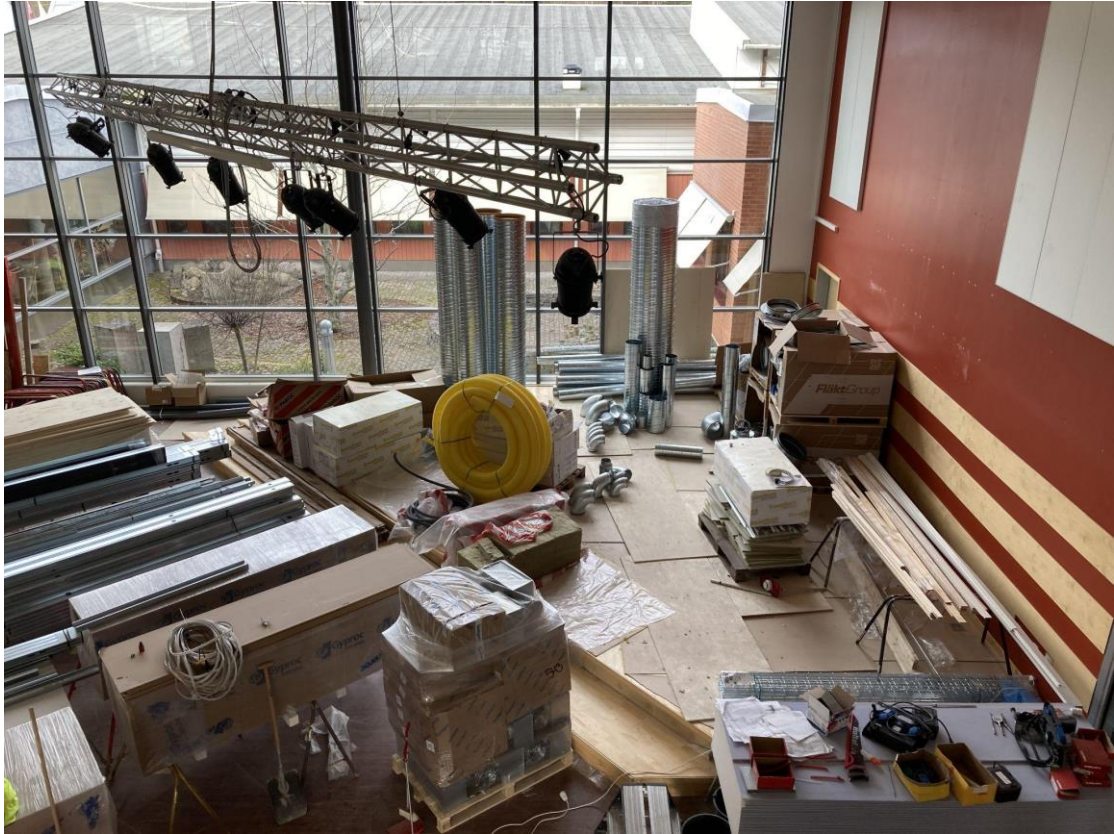
Figure 4.4 Material storage on site (Authors' own figure).
