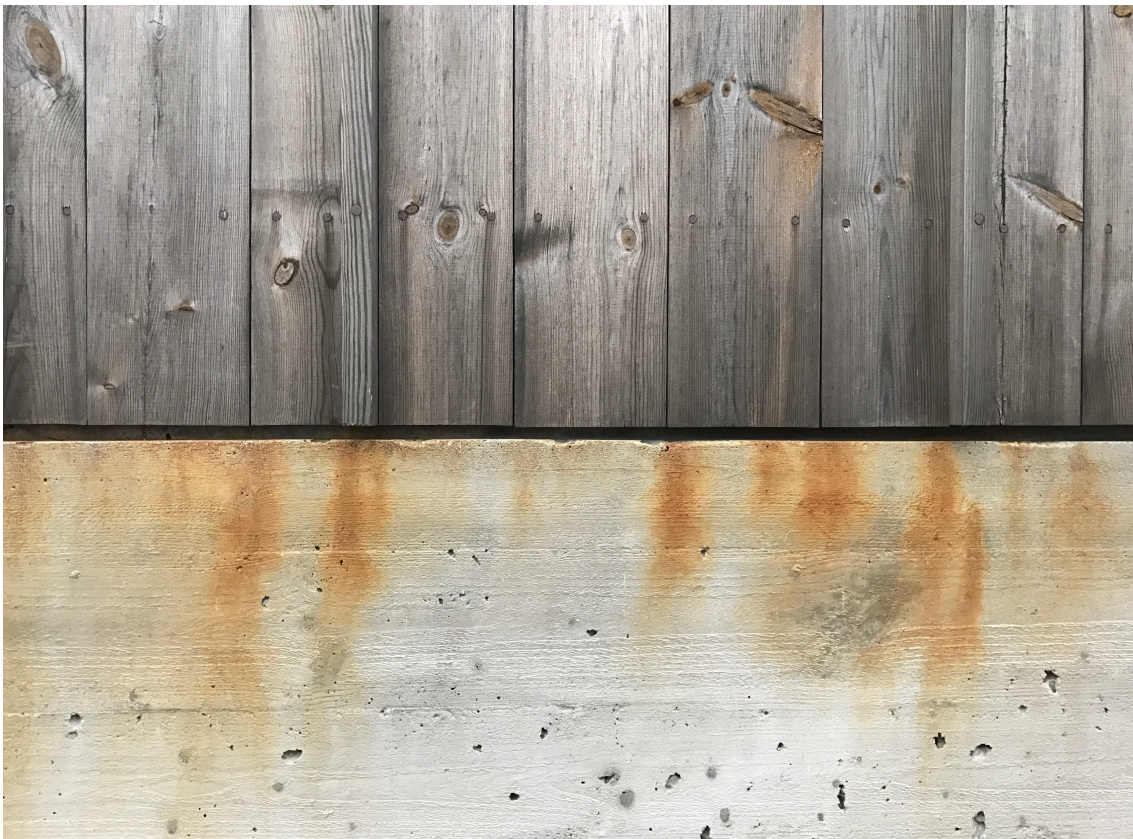
Figure A.1: Wooden panel treated with ferrous sulfate and concrete stained by runoff from the panel. Photo by the author.
