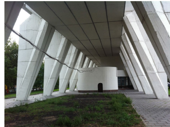
Building on pilotis
