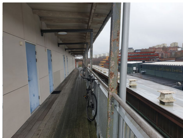
Building with external access to apartments
