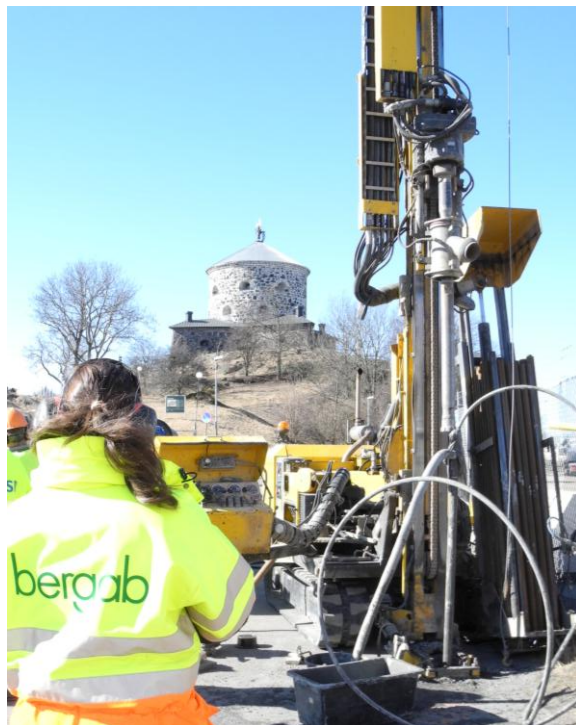
Figure 11 The hammer drill used at Skansen Lejonet
