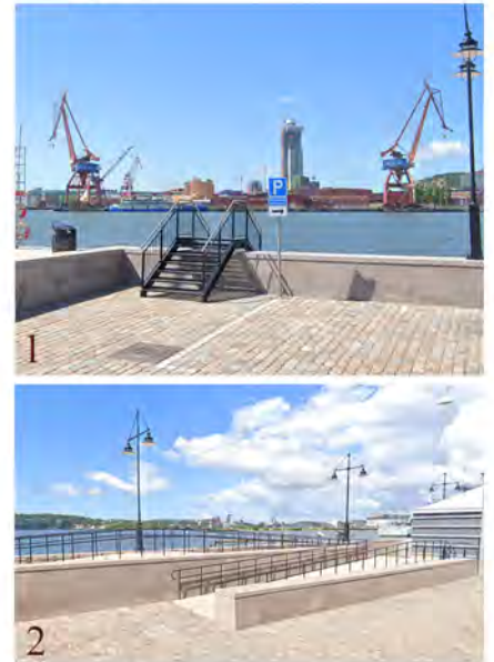
Floodproofing measurements taken from municipality
