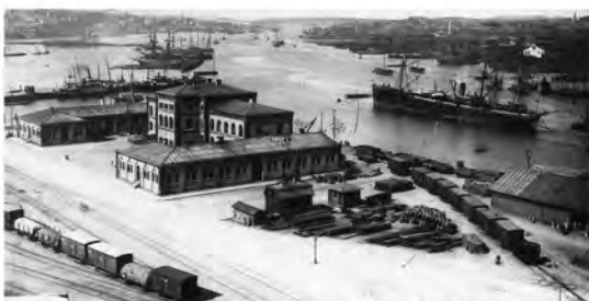
Fig 17. Exterior view of Tullpackhuset, Gothenburg.
