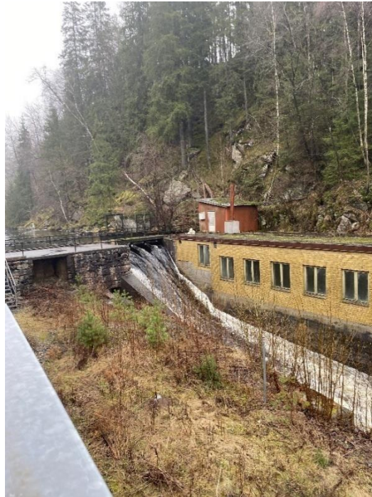
Figure 8. Hultafors regulating dam.
