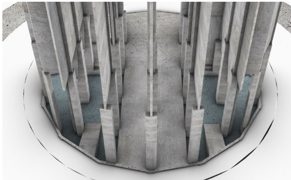
The floor is originally lowered and collects water into a floor pool around the raised isle.
