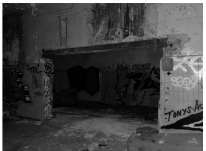
Vault rooms alterations
