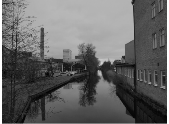
View canal south
