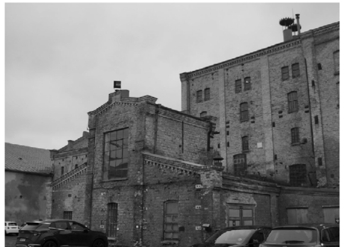
Main Brewery building
