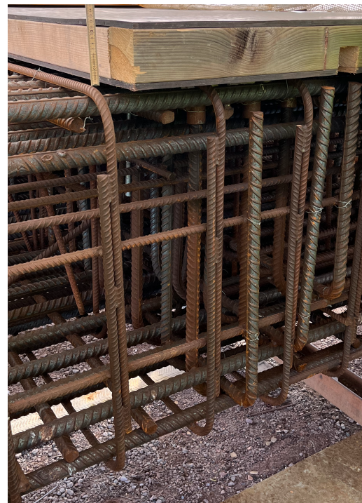
Figure 3.7: Wooden box covering the couplers at Korsvågen, Photo from Korsvågen 9/3-2022
