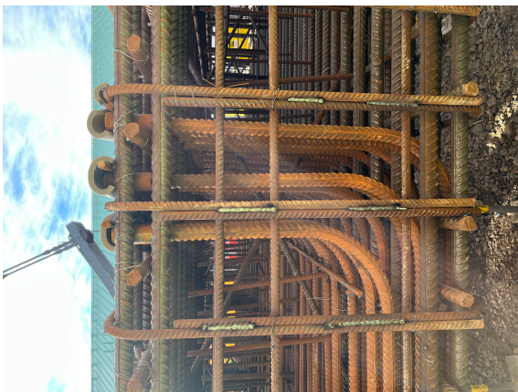
Figure 3.6: Reinforcement bars and couplers in reinforcement cage of a D-wall at Korsvågen, Photo from Korsvågen 9/3-2022
