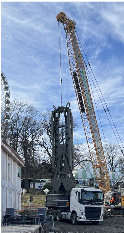
Figure 3.1: Machine used to excavate the trench of the D-wall, Photo from Korsvägen 9/3-2022
