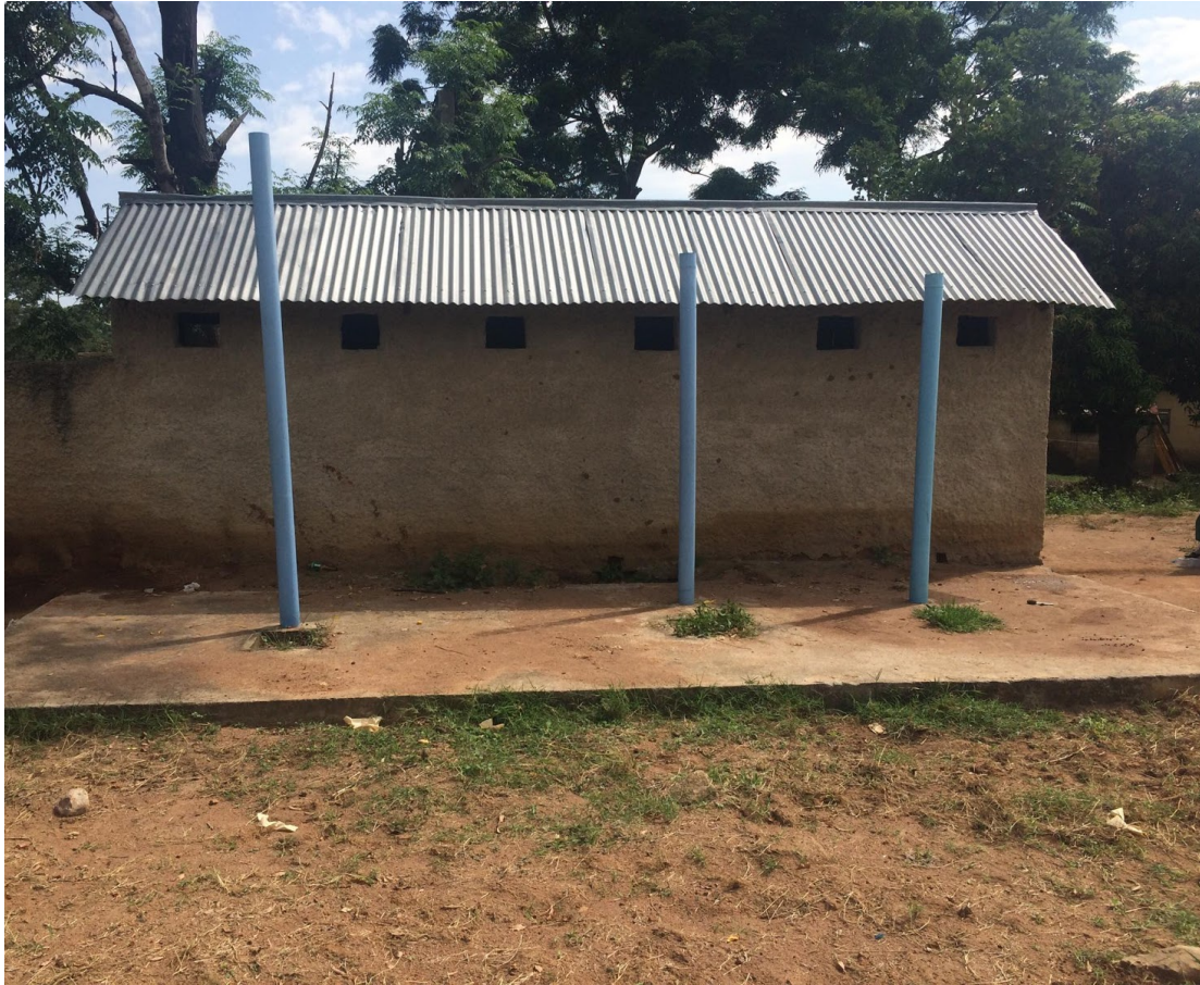
Figure iv. The back of the student toilets showing ventilation pipes.
