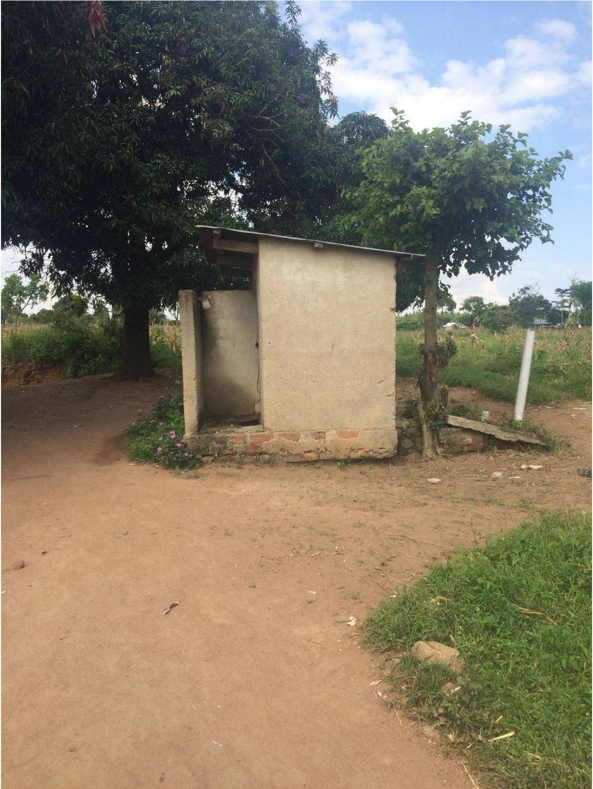
Figure iii. The teacher toilets seen from outside.
