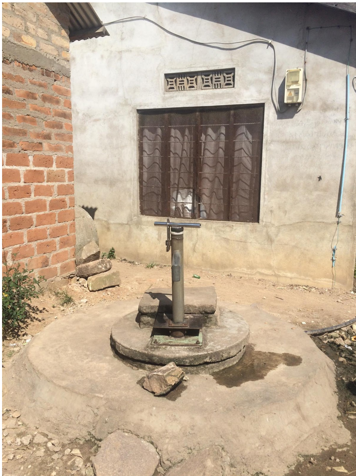
Figure i. Private well located in Bulyaheke.
