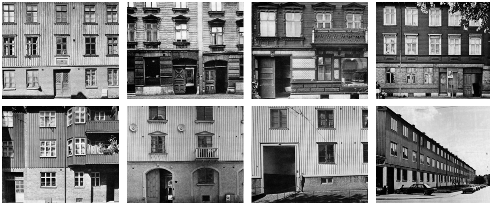
Fig 32-39: Facades of Landshövdingehus through time (Larsson & Lönnroth 1972)
