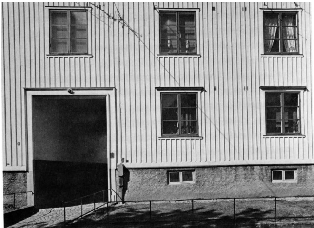
1928. Example of the facades from the modernistic era, with the wooden facades pulled down over the stone ground floor.
