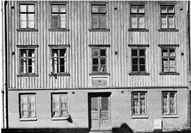
1875. Example of the simple facades with the ground floor covered in plaster.
