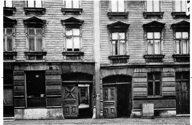
1891. Example of typical facades from the 1880s and 1890s with a rusticated ground floor and wooden ornamentation.
