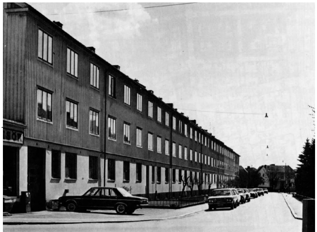
1935. Example facades from the modernistic area, with flat and simple wooden facades and plastered ground floor.
