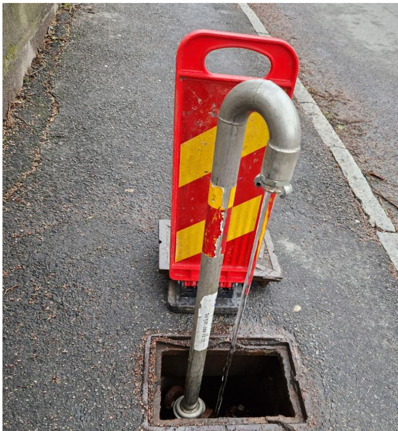
Figure 23: Upstream and Downstream fire hydrants where the water samples were collected.
