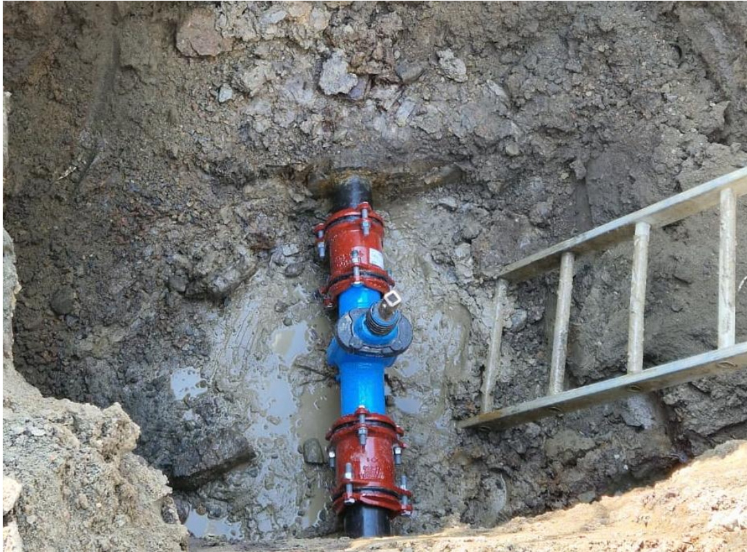
Figure 18: Leakage section after repair work
