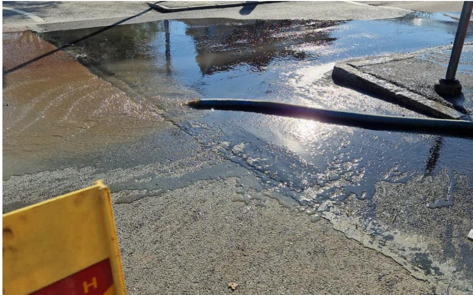
Figure 16: Flushing of excess water from the pit during the maintenance work
