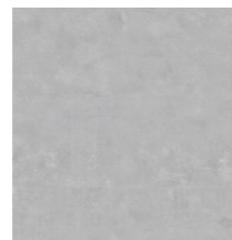
concrete, new floor
