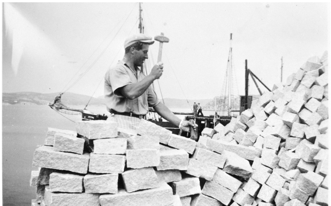
Fig. 5 Photograph from Bohusläns museum (UMFA53014:0021), depicting a stonemason cutting paving stone. Public domain.
