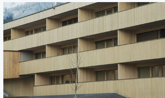
View of balconies
