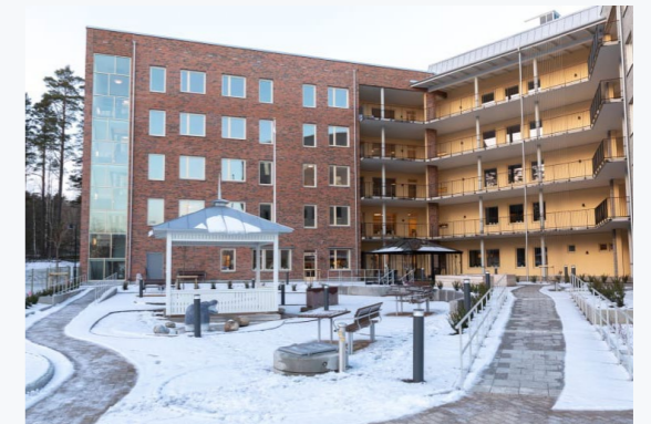
View of the courtyard
