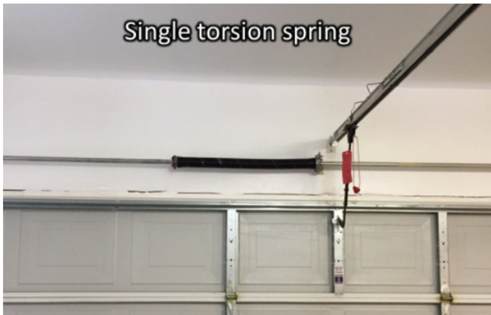
Figure 9: A garage torsion spring. This would reduce the force required to lift the truck axle by preloading the lift (Veteran Garage Door Service, 2022)
