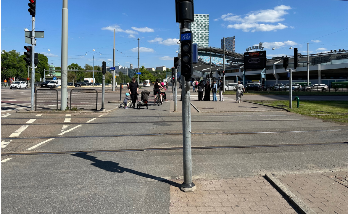
Figure 10. Traffic signal for cyclists in the south part of the intersection.
