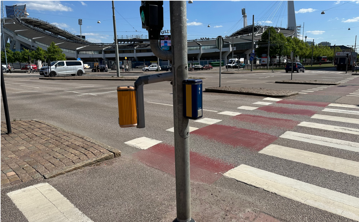
Figure 8. Push button detectors at part A of the crosswalk.
