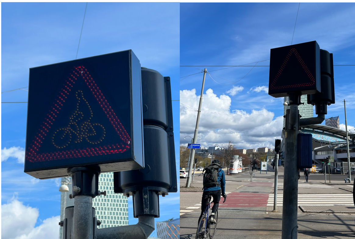
Figure 3. Warning for cyclists signs
